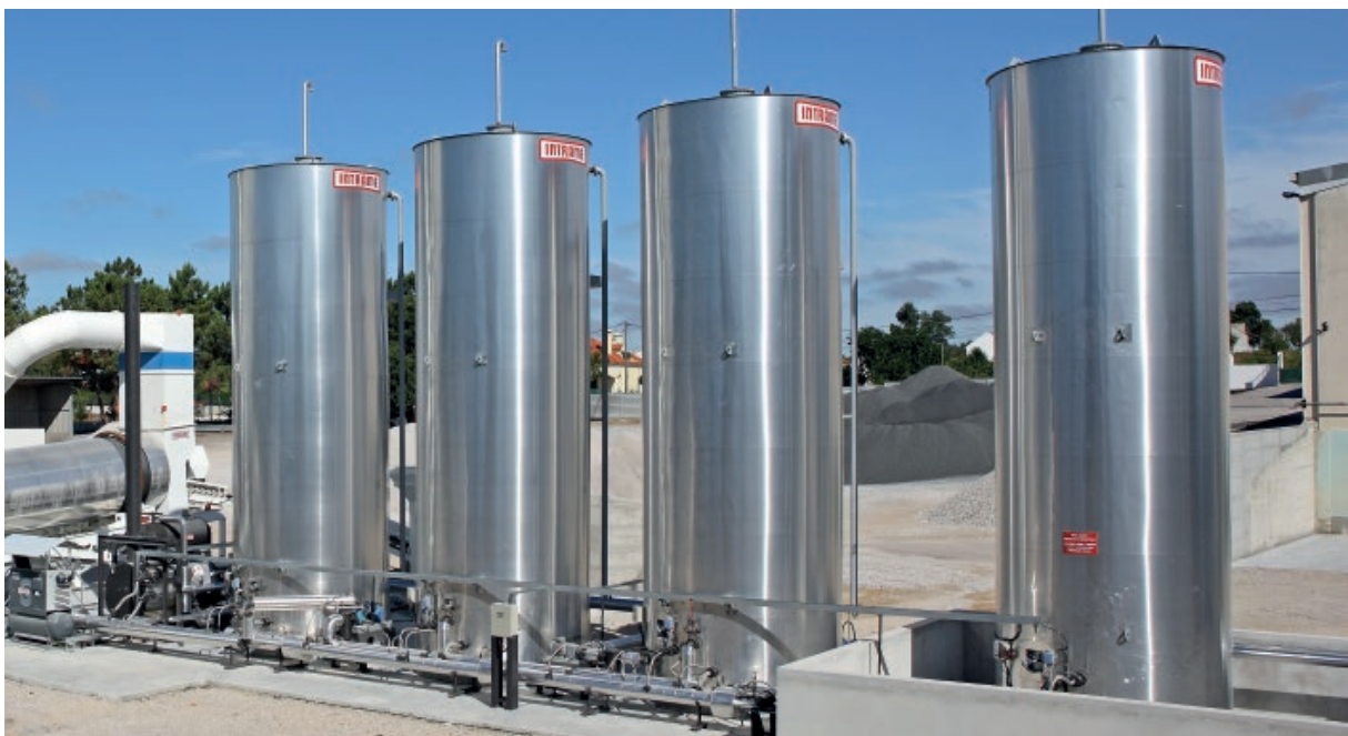
Vertical tanks heated by thermal oil.
