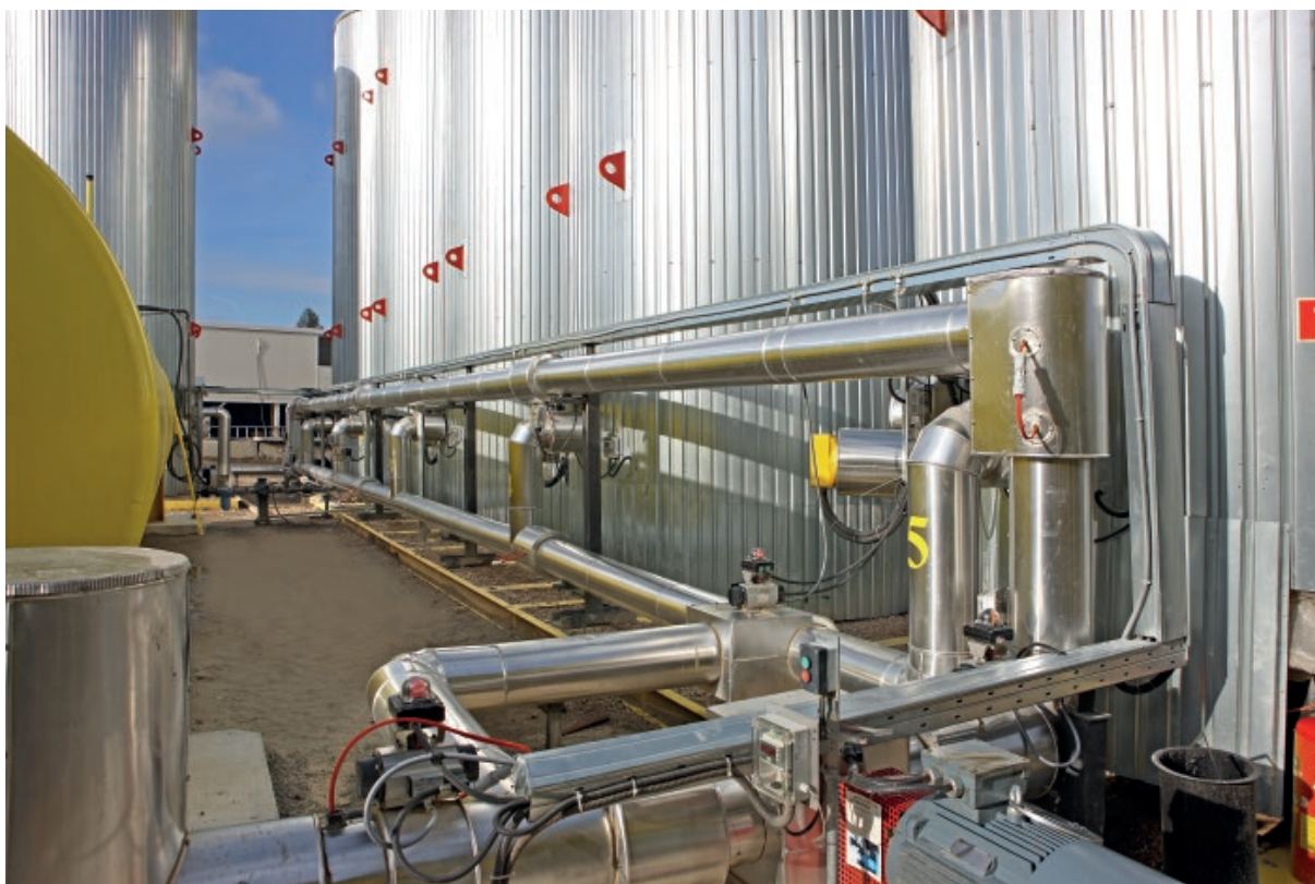
Electrically heated pipes in InNOVA 320 plant (Poland).
