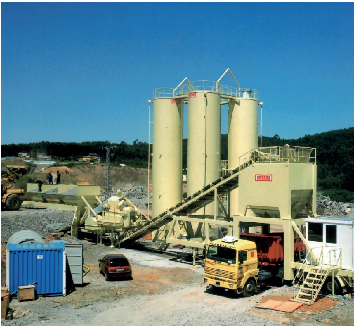
Soil stabilization plant GM-600.
