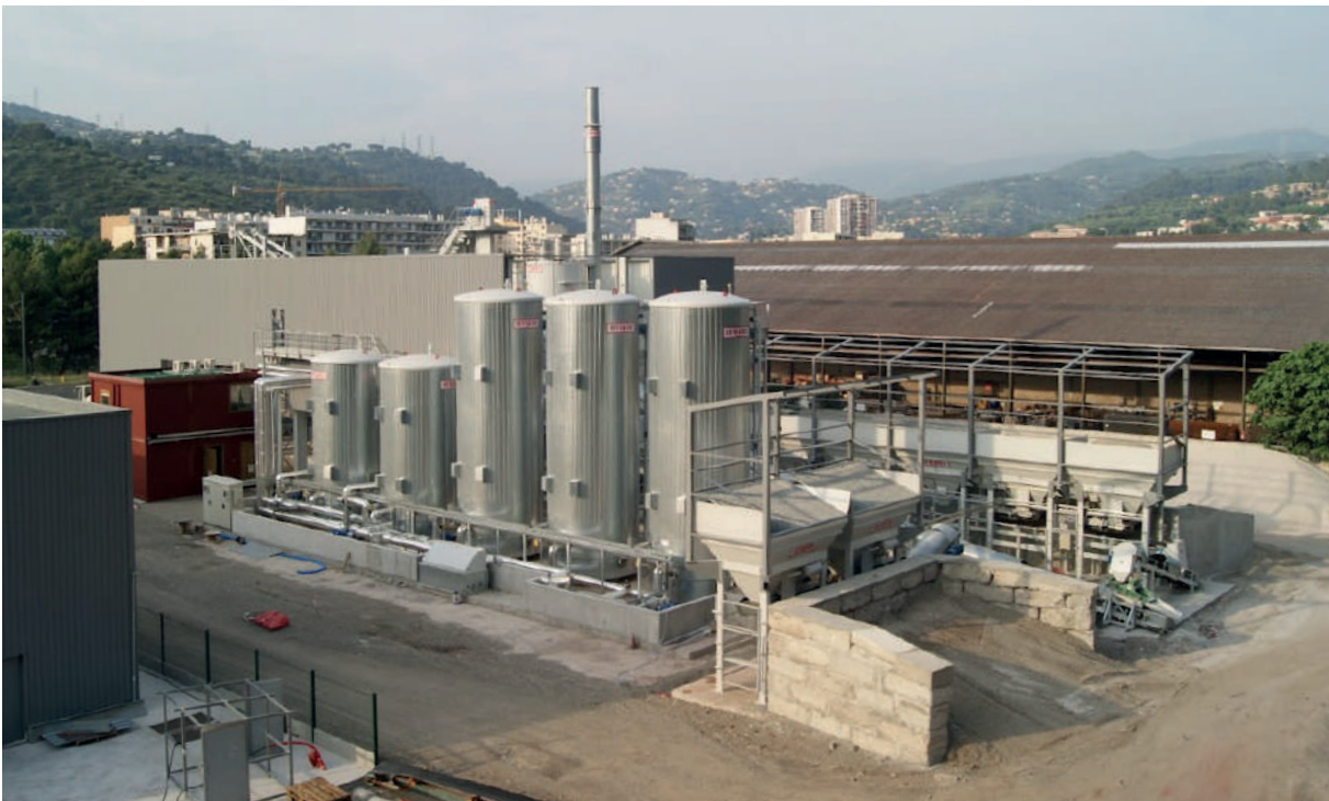
120 t/h asphalt plant with a special InNOVA-S mixing tower (without screen) partially enclosed in a metallic building. Equipped with cold process recycling system unloading in the mixer. Bitumen, emulsion and modified bitumen tanks electrically heated. 1.500 kg mixer. Installed in Nice (France).
