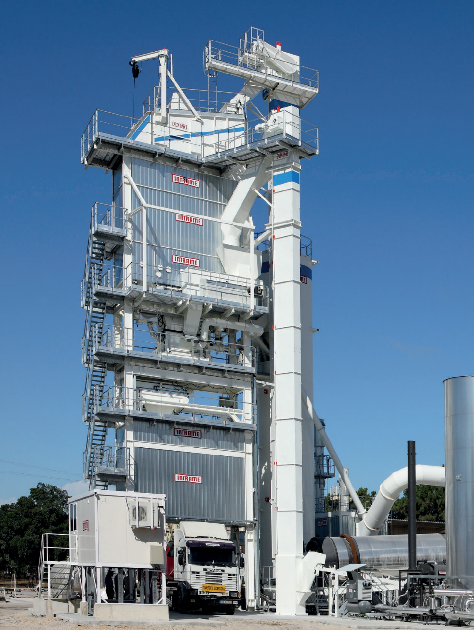
InNOVA-160 asphalt plant in Portugal
